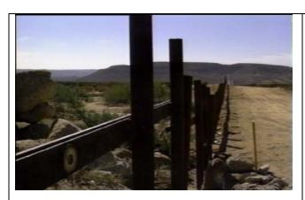
An example of this consideration for the environment is the modified vehicle barrier in the eastern San Diego county. This barrier impedes vehicle traffic while still allowing animal migration and water flow across the Mexico border.
